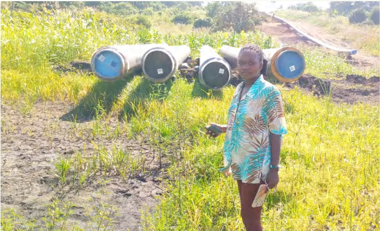
Oil feeder pipelines traversing community farmlands across Butimba in Kiziranjumbi sub county Kikuube district
