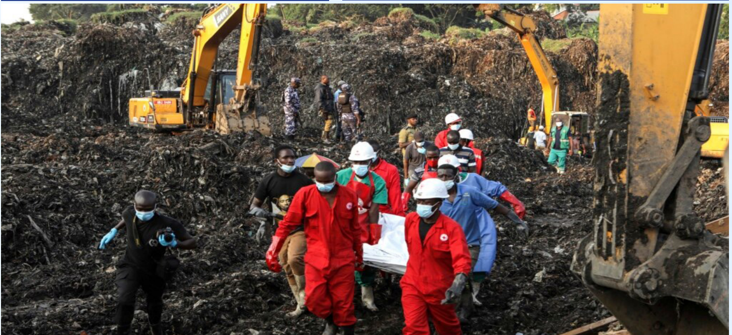
At least 35 people lost their lives following a devastating landslide at the Kiteezi landfill, the sole waste disposal site for the Ugandan capital, Kampala. Photo by AP
