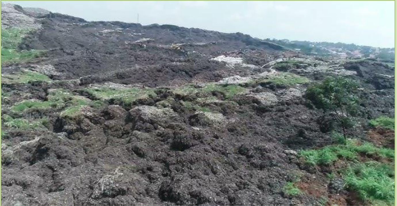
The collapse of landfill in Kiteezi, Kasangati Town Council, Wakiso District
